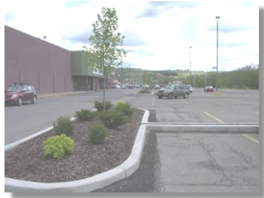
The installation of curbed planting beds in the Riverside Plaza parking lot enhances the character of the development while improving traffic flow. Medians such as these should be required as part of any site plan review for future commercial projects.
